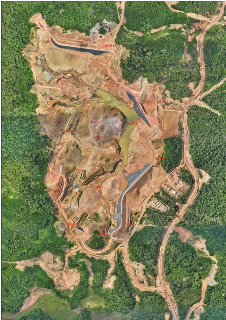
TIFF showing UAV survey of TSF.
