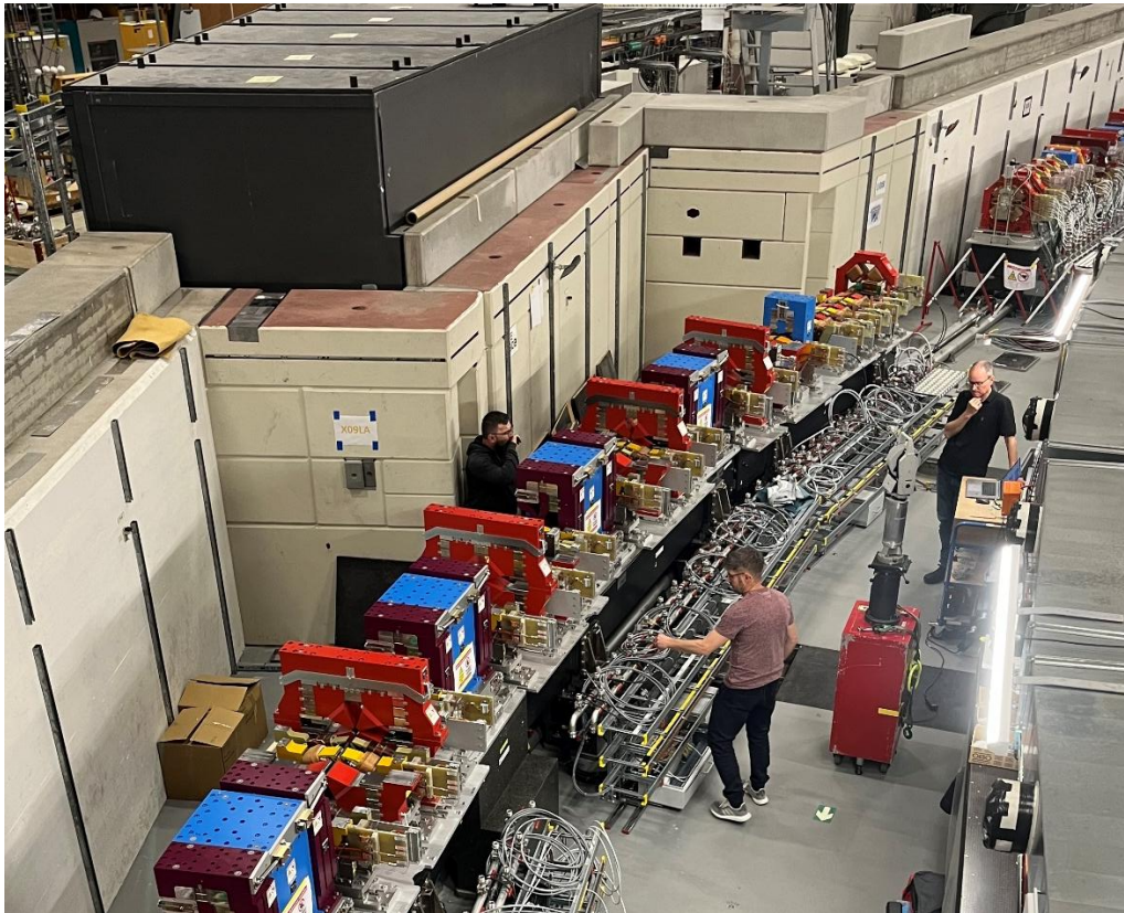
Figure 4. Initial Alignment of the SLS 2.0 Girders
