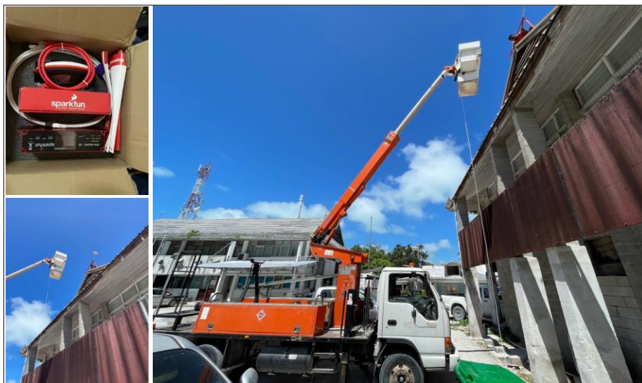
Figure 7: CORS bracket installation & SparkFun equipment — SparkFun kit (top left), antenna install (bottom left) and CORS bracket installation (right)
