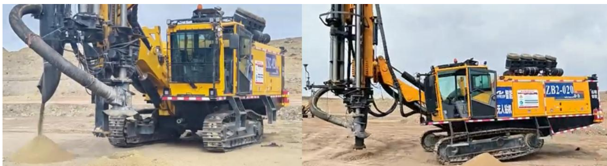
Figure 11-Application at Job Site
