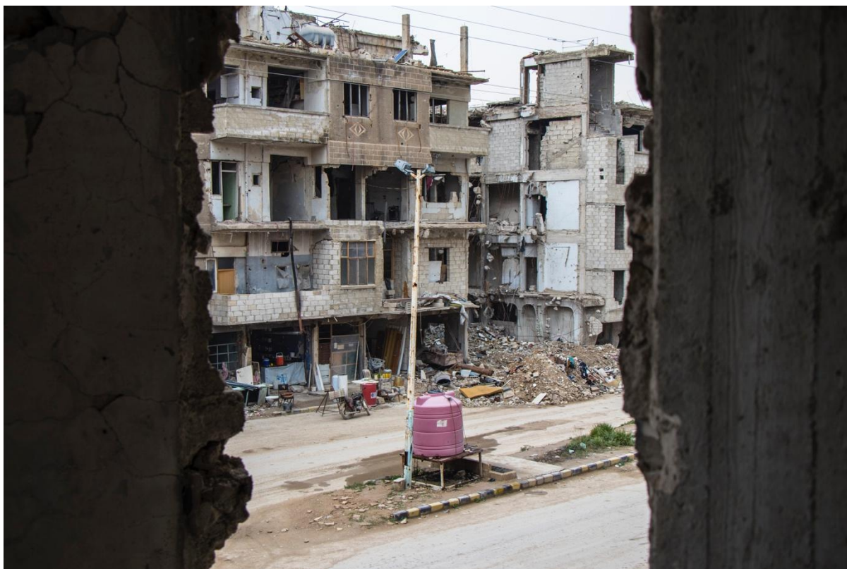
Figure 1 war-damaged residential buildings in Harasta, eastern Ghouta, Syria. Source: International Committee of the Red Cross (ICRC), ICRC Visual Archive (n.d.)
