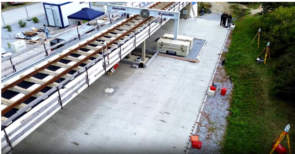
Arrangement of the loading portal and total stations for control measurements (right)
