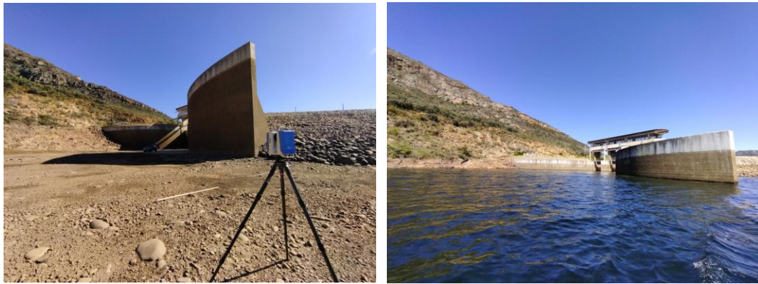
Figure 2. left TLS Scan at 50% capacity; right second MBES survey at 85% capacity
