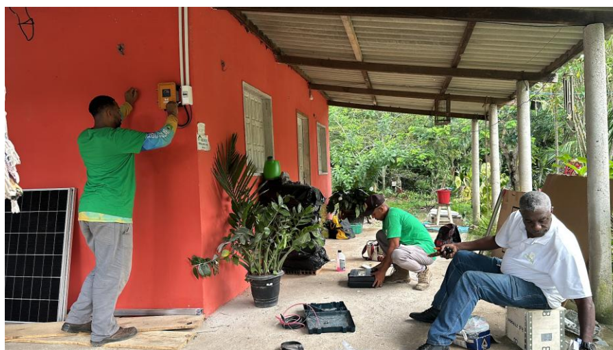
Figure 4 - Installation of photovoltaic energy panels
